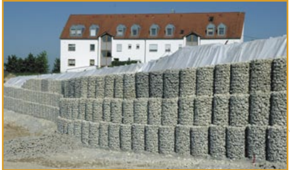
Embankment stabilization in Reichenschwand: FERRONDO® adapts to any kind of terrain
