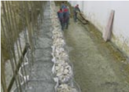
The lower layers are partially filled with concrete.
