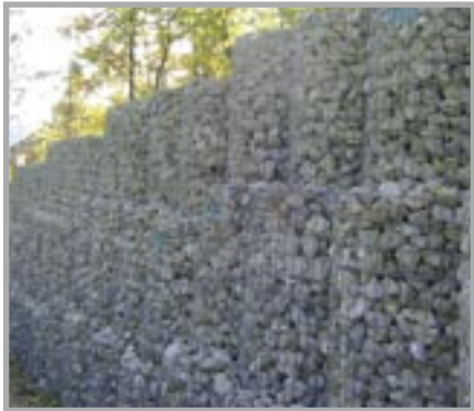
Slope stabilization filled with natural stone
